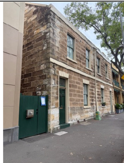
Figure 4.0, Easement entrance to subject property at 125A Kent Street, with 125 Kent Street on RHS, AW 23.02.26
